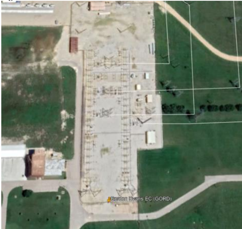
Figure 33 – Gordon Evans 138kV Substation
